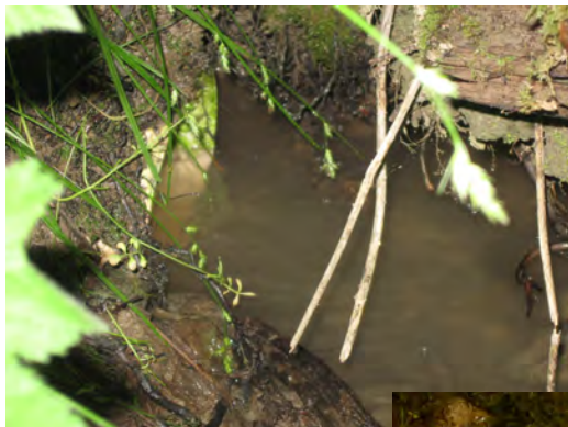
Photo 11. Surface drainage in ditch
