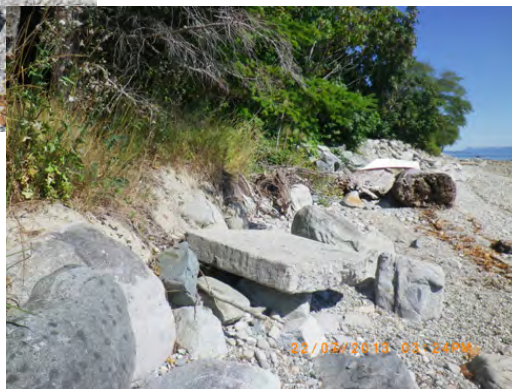
Photo 17. Erosion of unprotected shoreline
