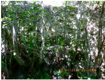
Photo No. 5 Area of slump, Atrevida Road
