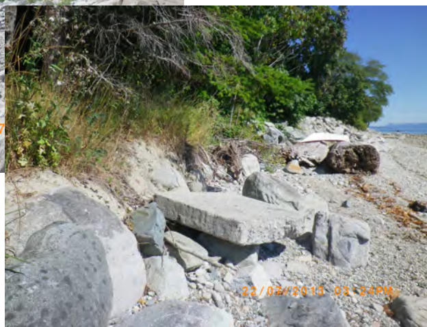
Photo 8. Shoreline erosion , Atrevida Rd.
