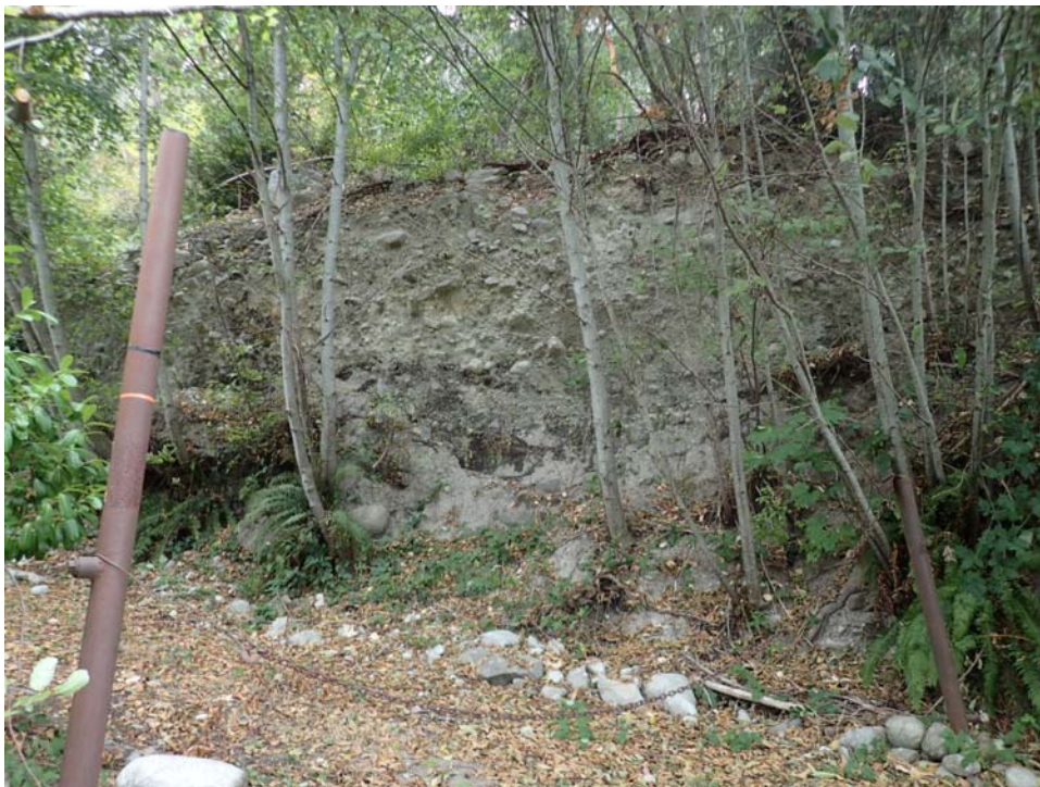
Steep cut with seepage near Atrevida Road.
