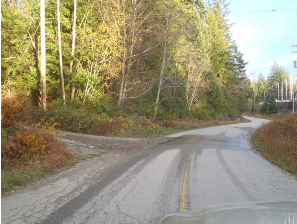
Uncontrolled drainage on Finn Bay Road
