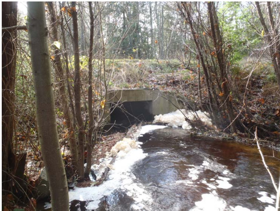
Winter flows with log blockage at culvert entrance on Kelly Creek (November 2017).
