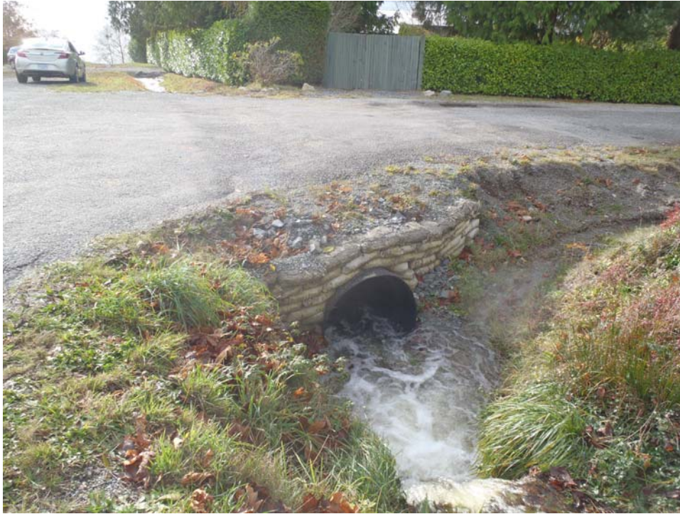
Flowing ditch on Pine Tree Road. Residents indicated that the flow at the time of the photo was relatively
