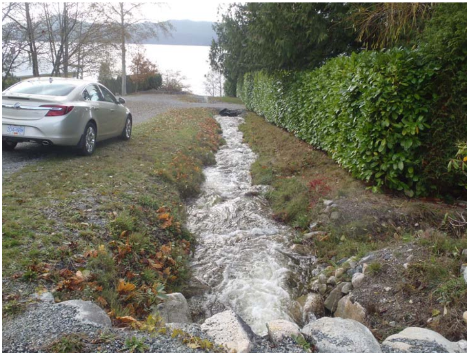
Creation of new concentrated flow path along rip rap lined channel on Pine Tree Road
