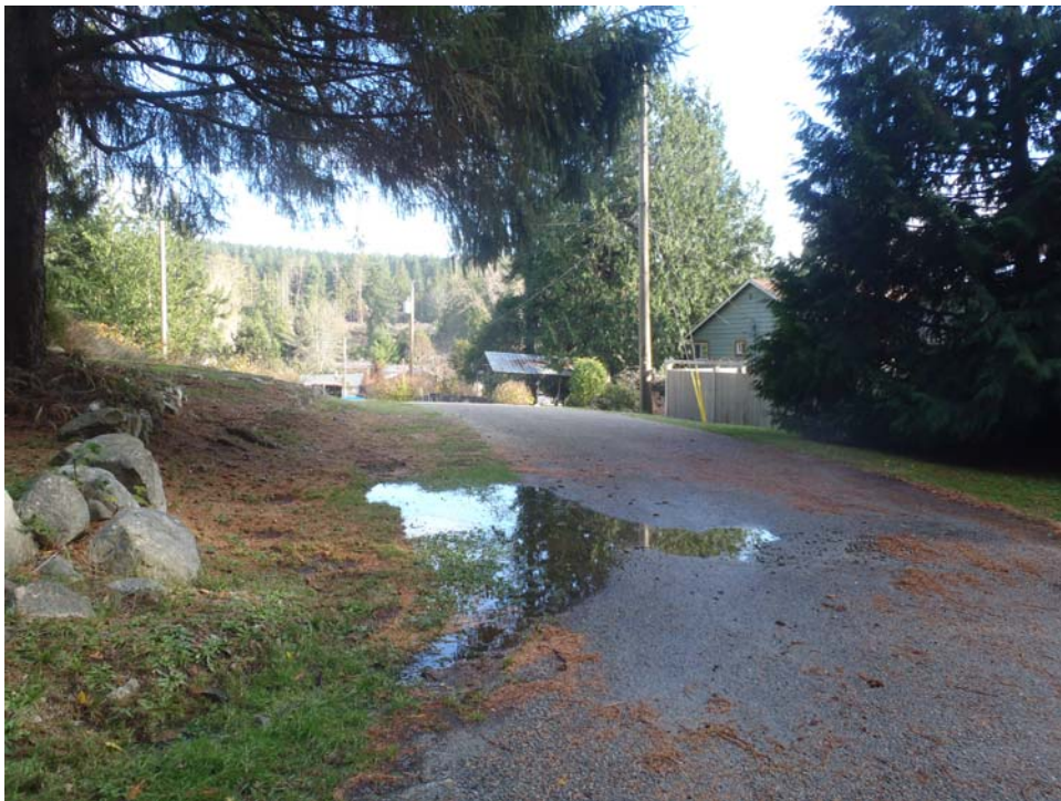
Standing water at Arbour Drive.
