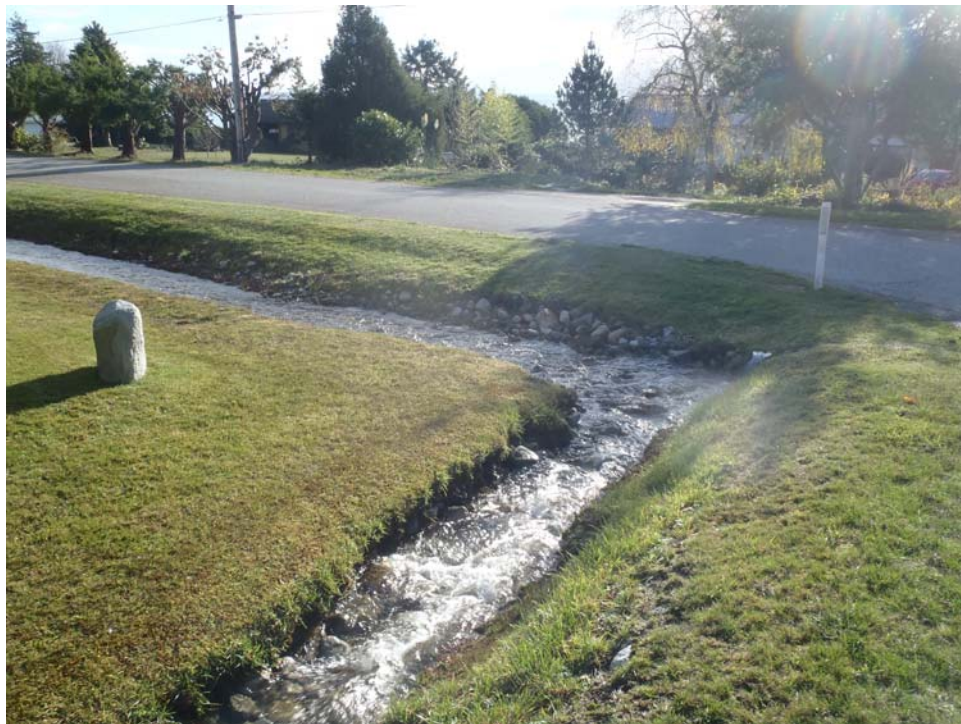
High flow in ditches along Victory Road.
