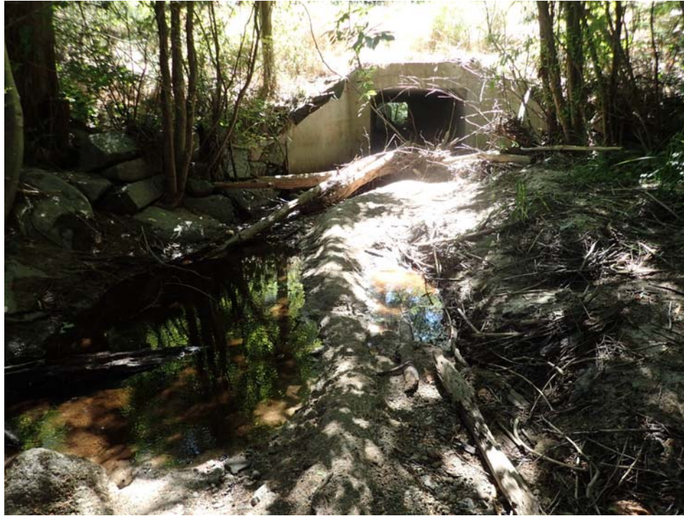
Build up of sediment and debris at Kelly Creek Culvert under Highway 101 (August 2017).
