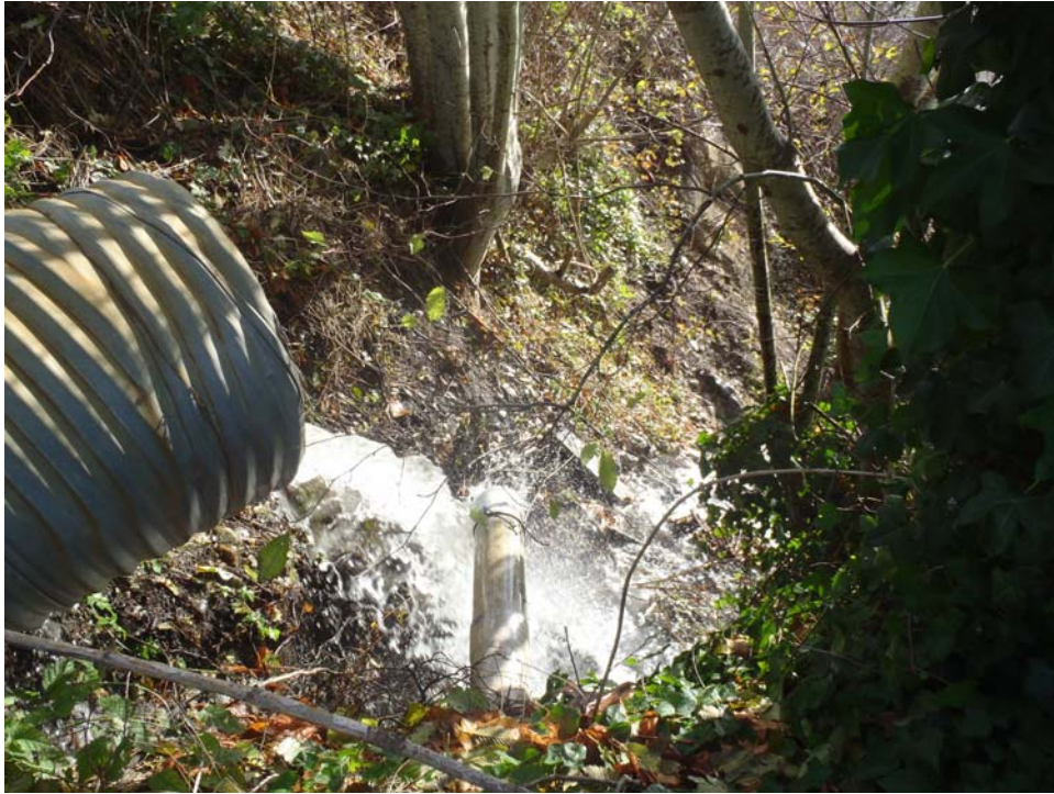
Discharge eroding the bluff at Reave Road
