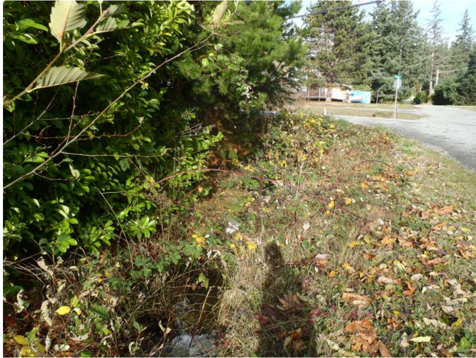
Typical unmaintained ditch/culvert outlet.
