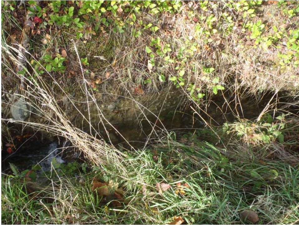
Ditch along Reave Road.
