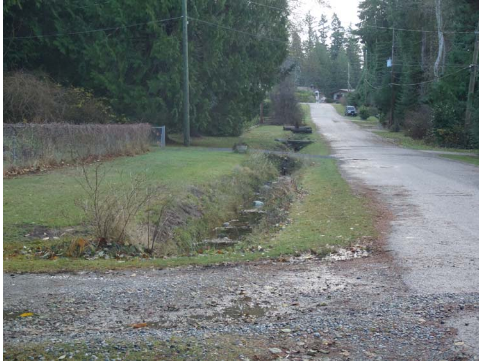
Example of driveway culverts and ditches along Traff Road.
