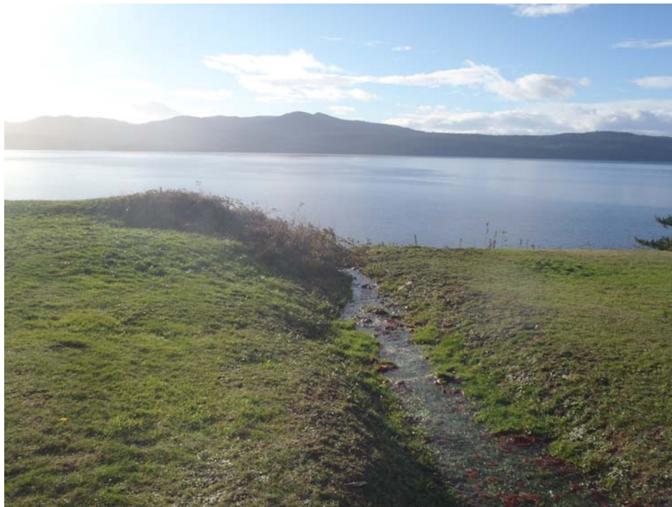
Ditch spilling water onto eroded bluff at Fleury.
