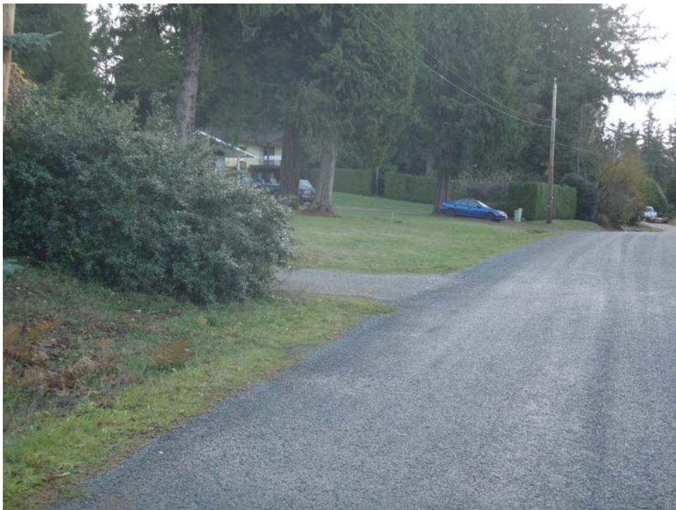
Filled in ditch on Myrtle Point Road, causing drainage flowing onto down slope properties (8611/8612).
