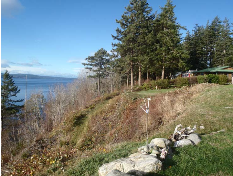
Eroding bluff at Fleury Road ditch outfall.
