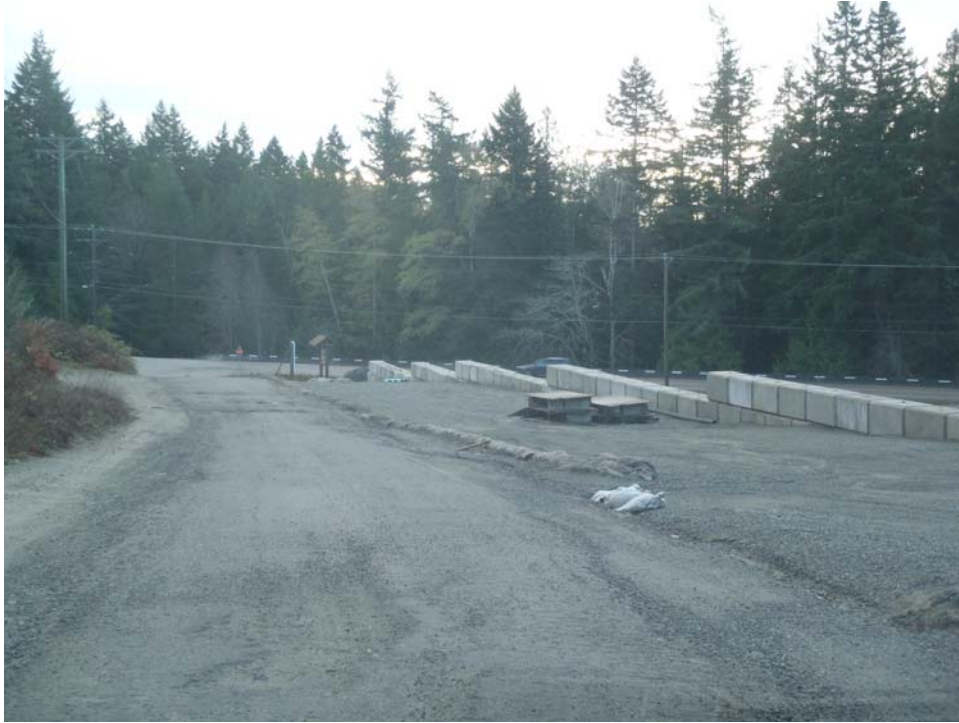
Lack of ditches at Stevenson Road. Evidence of road erosion.
