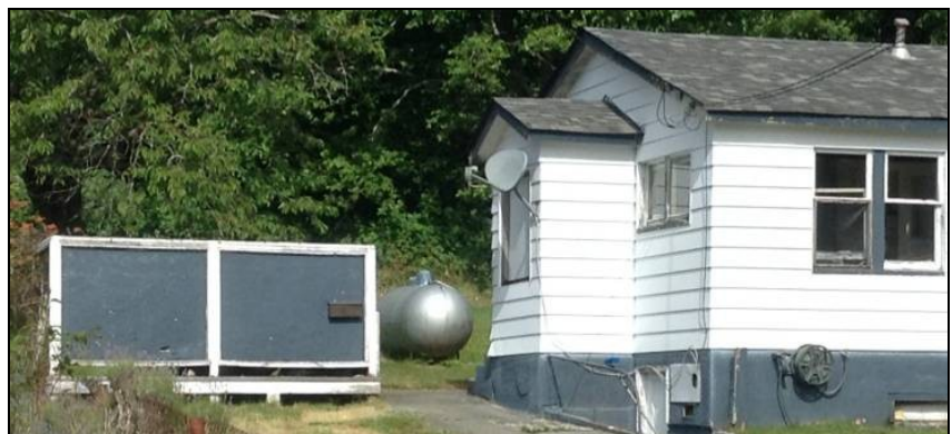
Figure 7. Example of a combustible material (propane tank) stored within 10 m of a residence.
