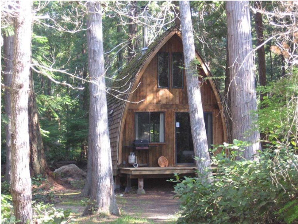
Figure 8. Photograph showing no setback from forested vegetation and unrated roofing material present on some homes within the wildland urban interface.
