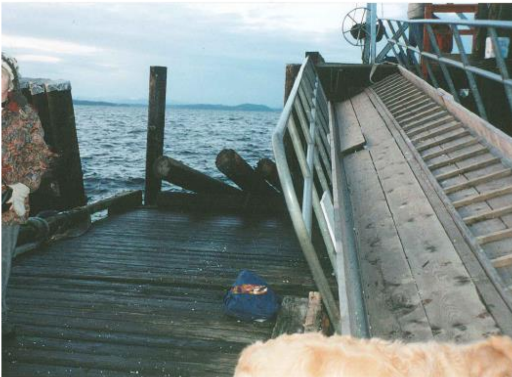
The two photos show the Savary wharf damage (photos by Lund Water Taxi Service).
