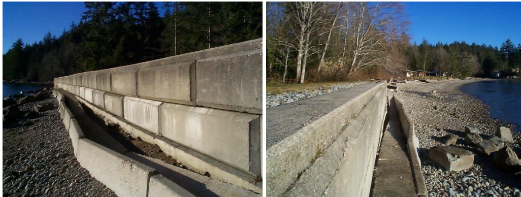
Photographs: View of storm damage to the breakwater at Saltery Bay Provincial Park, located west of the Saltery Bay ferry terminal
