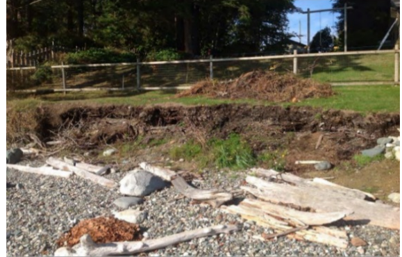
Figure 5-2. Example of coastal erosion in PRRD.
