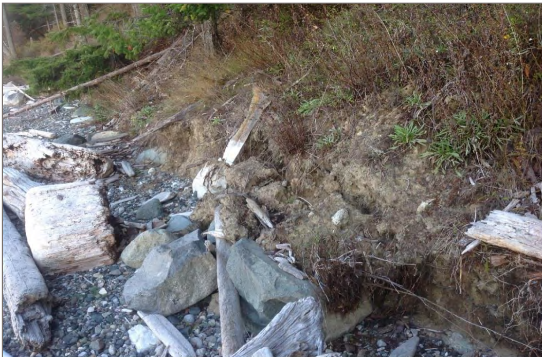
Photo 12: View of coastline erosion to the west of Gillies Bay, along the section of coastline between the cable TV tower and the "Sand Banks" area. (Photo taken October 2016).
