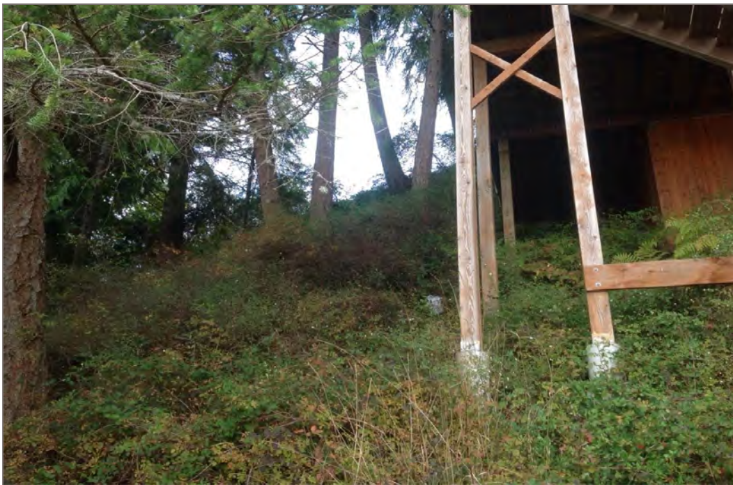
Photo 10: View of coastal escarpment along east side of Gillies Bay. Curved / tilted tree trunks indicative of slope creep and potential slope instability. (Photo taken October 2016).
