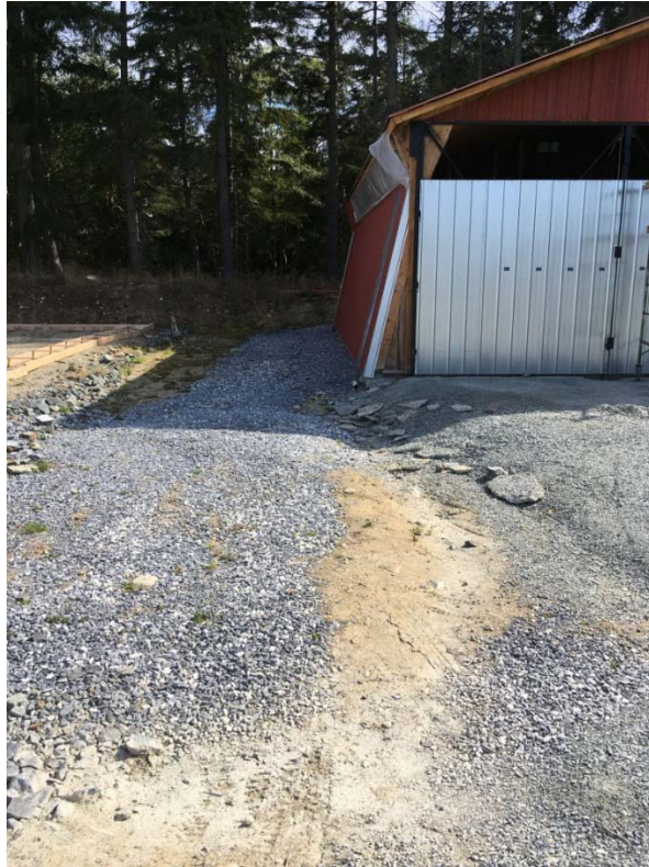
Photograph 3: Roof drainage causing minor erosion and wet season ponding
