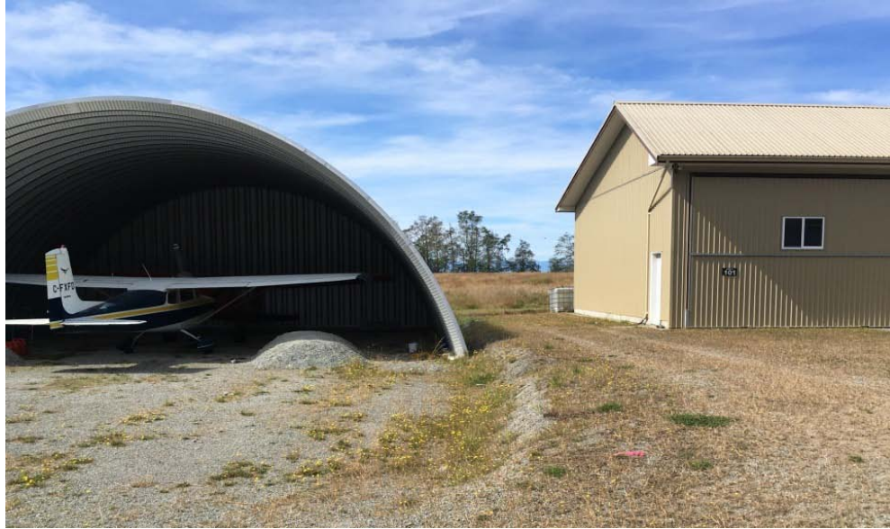
Photograph 2: Mismatching surface grades between adjacent hangar lots
