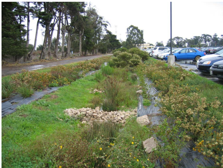
Photograph 4: Example of bioswale and rock check dam for sediment and erosion control
