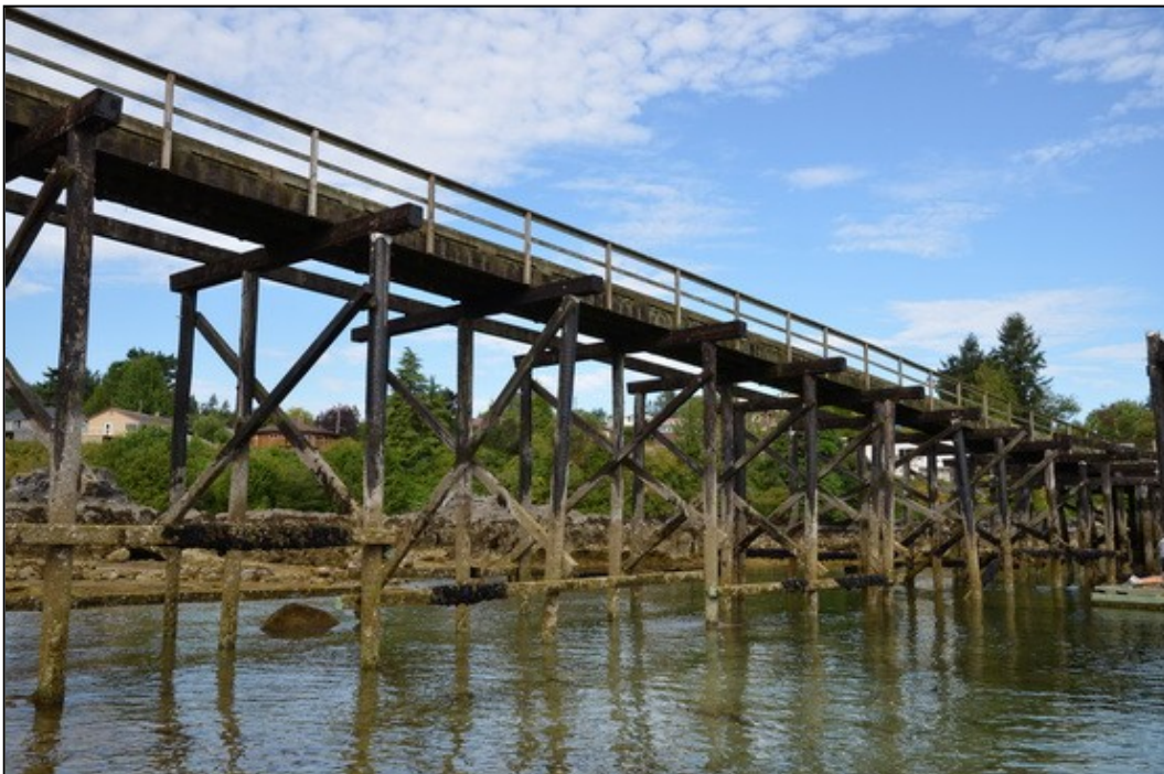
PHOTOGRAPH 4. Typical configuration of the approach sub-structure with piles, cross-braces, walers, caps, stringers and decking.
