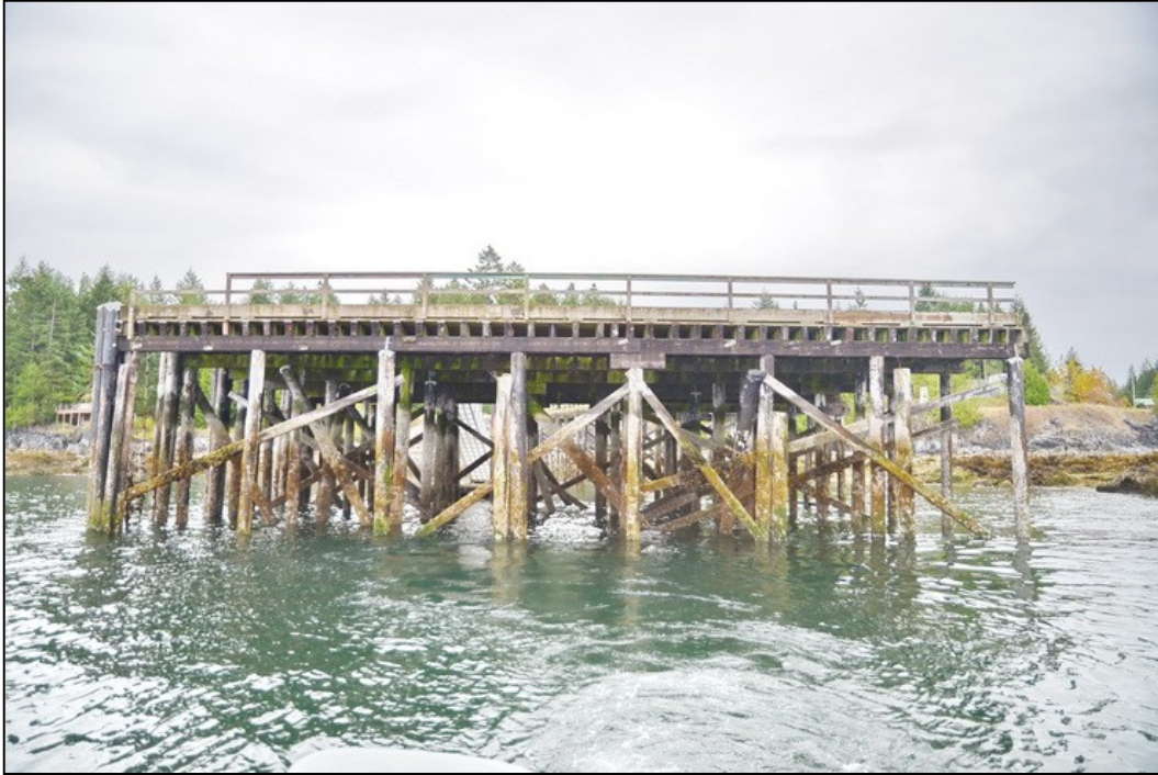
PHOTOGRAPH 5. West side of the wharfhead (Bent 24) showing piles, bracing, caps, stringers and railing.
