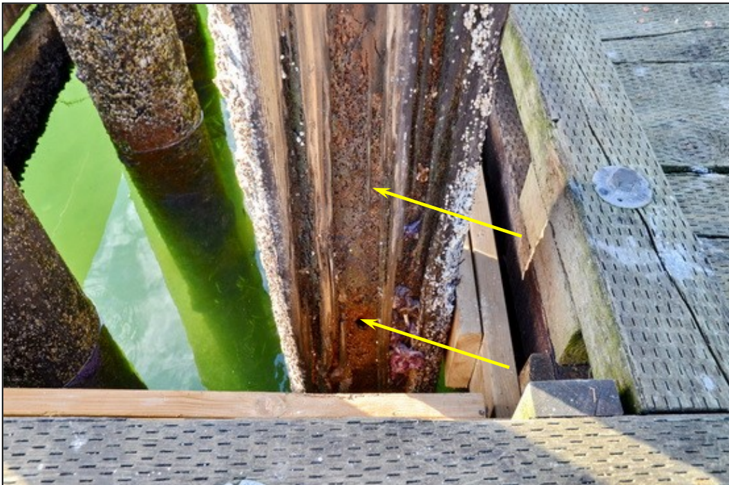
PHOTOGRAPH 22. Float anchor pile (East Cluster SW corner) has a combination of abrasion and marine borer damage. This pile will likely require replacement within the next 3 to 5 years
