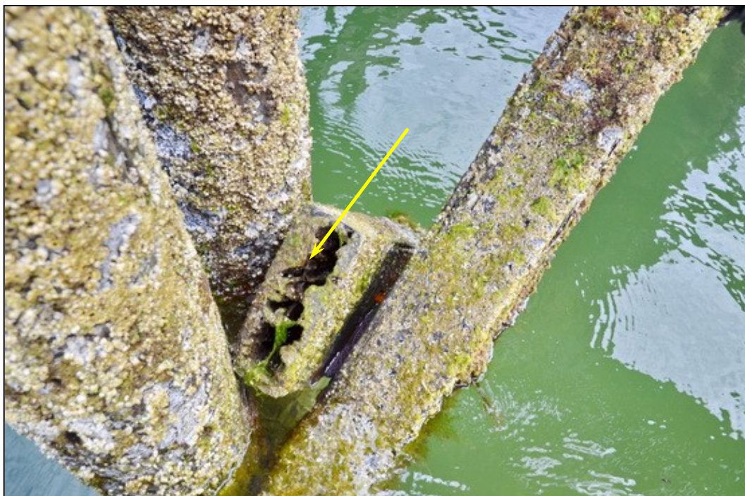
PHOTOGRAPH 12. Heavy marine borer damage to a spacer block between the cross-brace and the pile in the approach.
