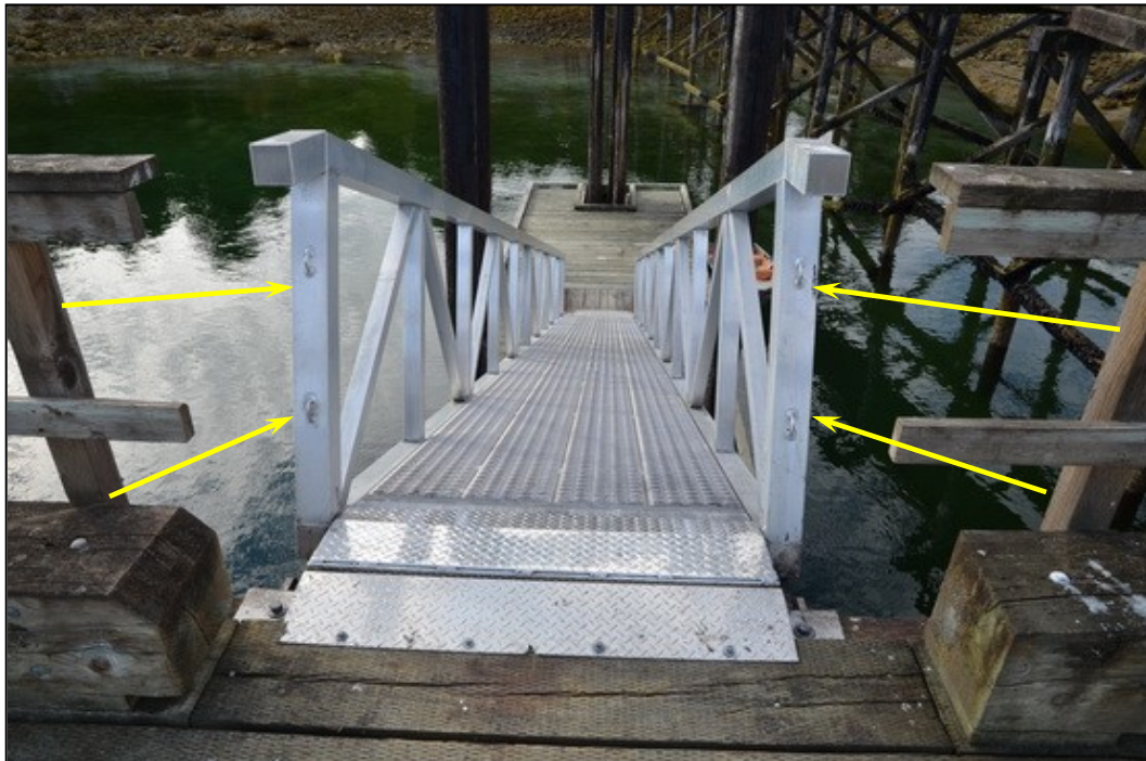
PHOTOGRAPH 18. Eyes are present on the gangway to secure safety chains to the posts around the wharfhead. Chains are missing.
