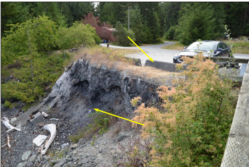
PHOTOGRAPH 24. Erosion of the bank along the north side of the approach creates the potential for a slope failure. Concrete barriers are located along the top of the slope. The area should be armoured with rip-rap to prevent further erosion.
