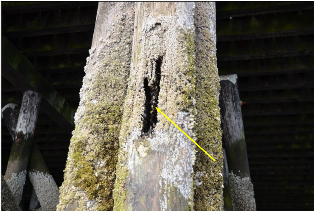
PHOTOGRAPH 16. Heavy marine borer damage to one of the fender piles along the north side of the wharfhead.
