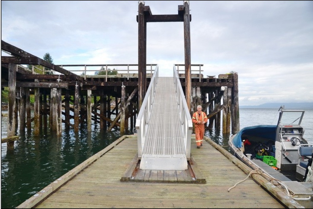
PHOTOGRAPH 7. Aluminum gangway that extends from the wharfhead down to the float.
