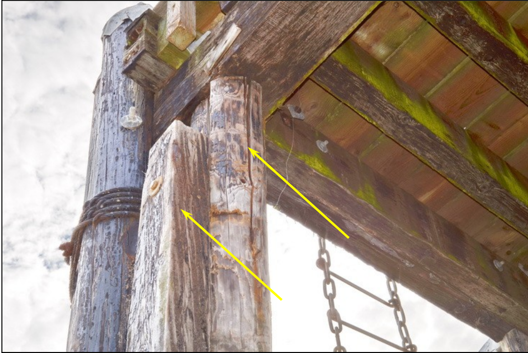
PHOTOGRAPH 15. Mechanical impact damage to Pile 24 – H in the wharfhead. The pile is badly split, and the associated cross-brace has failed.
