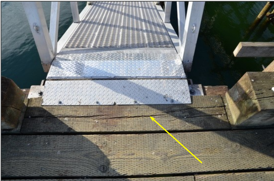
PHOTOGRAPH 14. Deck at the top of the gangway is badly split and is recommended for replacement.
