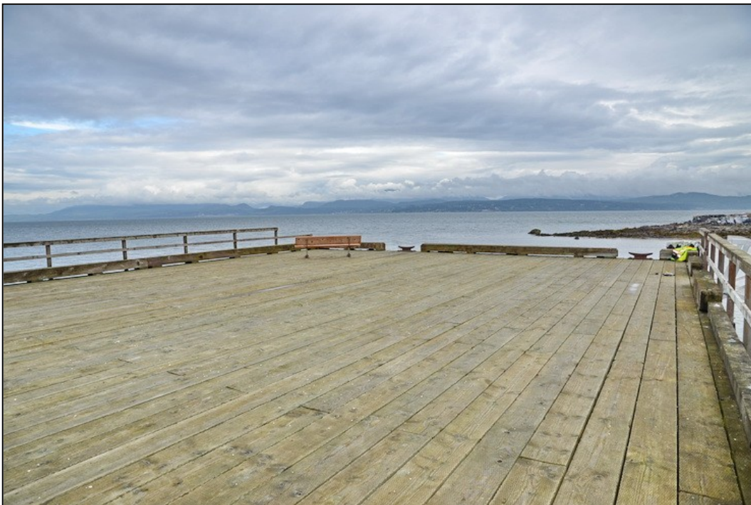
PHOTOGRAPH 6. Deck of the wharfhead looking north. The north side does not have handrails.
