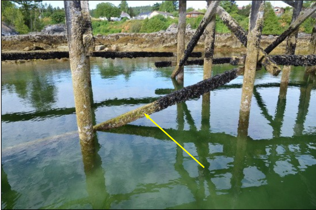
PHOTOGRAPH 13. Failed horizontal waler along Row C in the approach.
