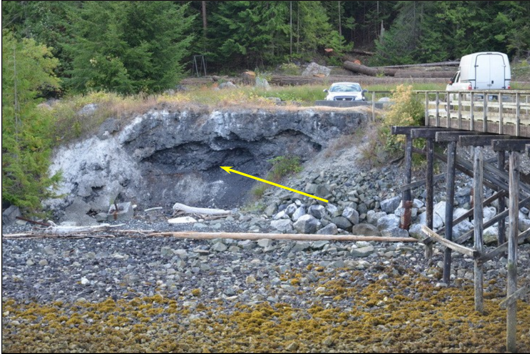
PHOTOGRAPH 23. Erosion of the bank along the north side of the approach creates the potential for a slope failure.
