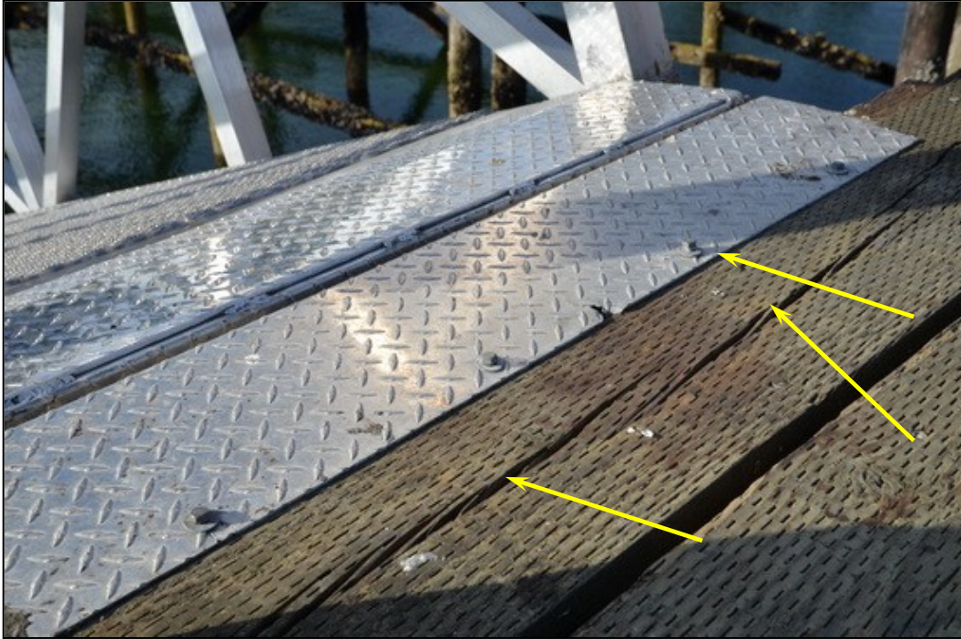
PHOTOGRAPH 19. Bolts securing part of the upper transition plate are loose. Mounting timber is also split.
