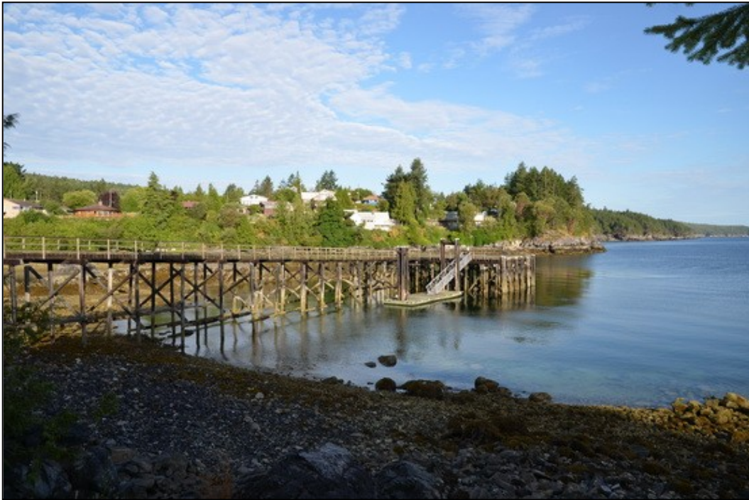
PHOTOGRAPH 1. Van Anda Dock, Texada Island. Approach, Wharfhead and Float.
