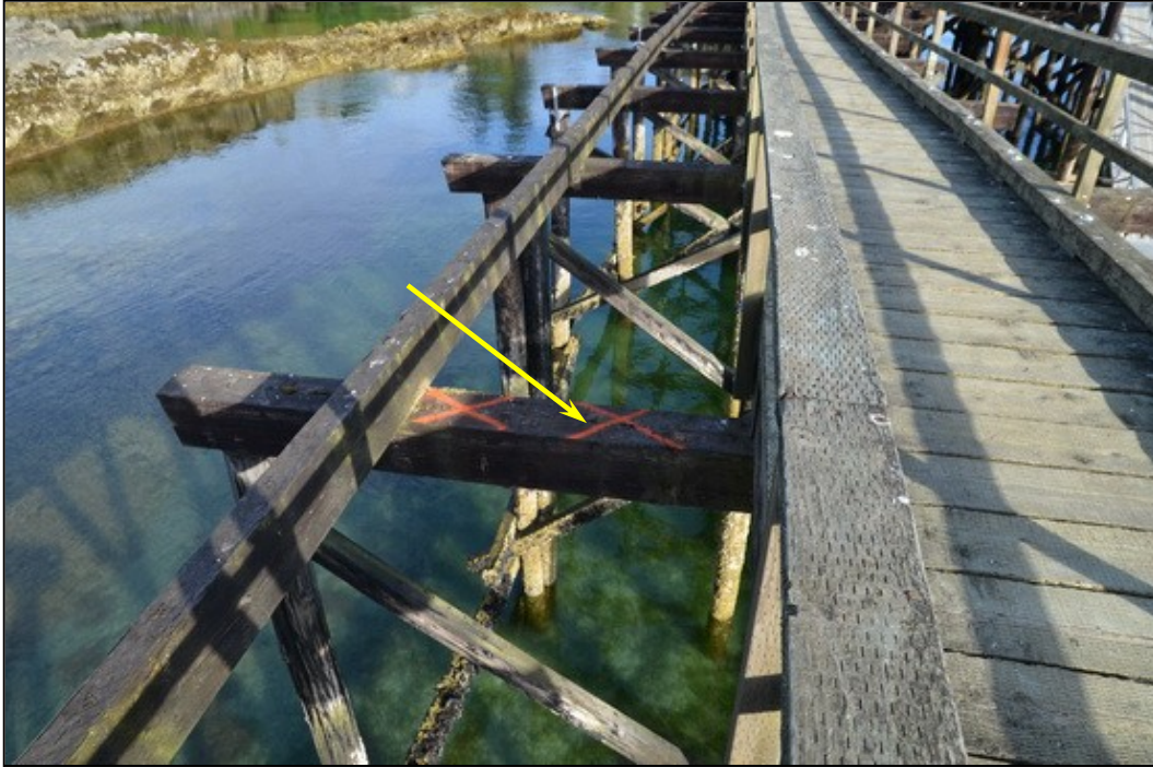
PHOTOGRAPH 9. Cap located at Bent 11 in the approach has heavy fungal damage from Row A (left) to Row B (middle).
