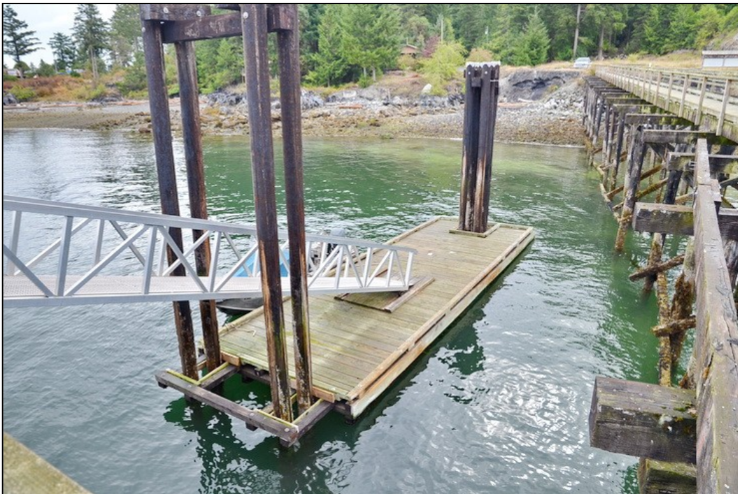
PHOTOGRAPH 8. Float and float anchor piles.
