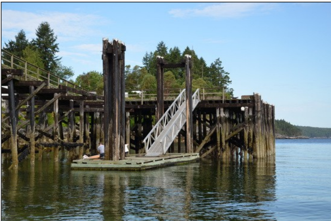
PHOTOGRAPH 2. Float and Float anchor piles along with gangway at the northeast side of the wharfhead.
