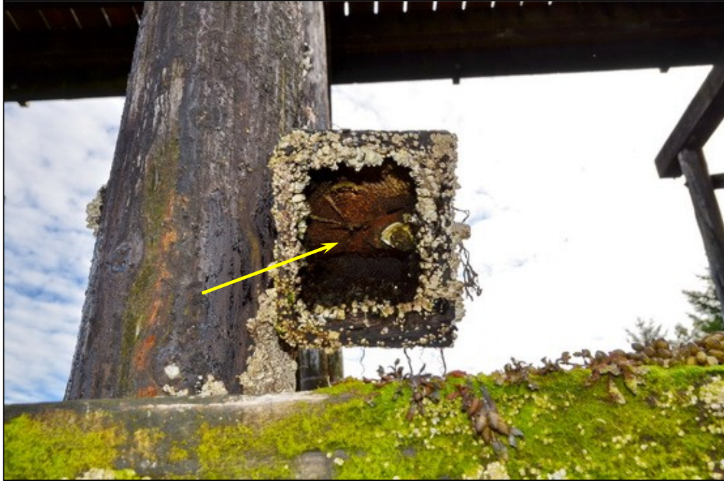
PHOTOGRAPH 11. Marine borer damage in the lower end of a cross-brace in the approach. Damage extends up to the attachment bolt.
