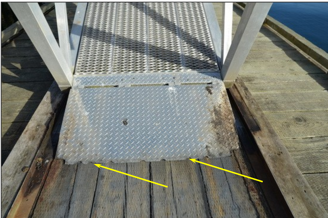
PHOTOGRAPH 20. The lower edge of the lower transfer plate abrades with the pad that supports the sliders and ramp guides. It remains functional.
