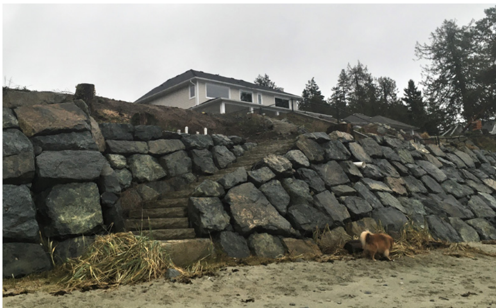
▲ Shoreline revetment for new residential development
