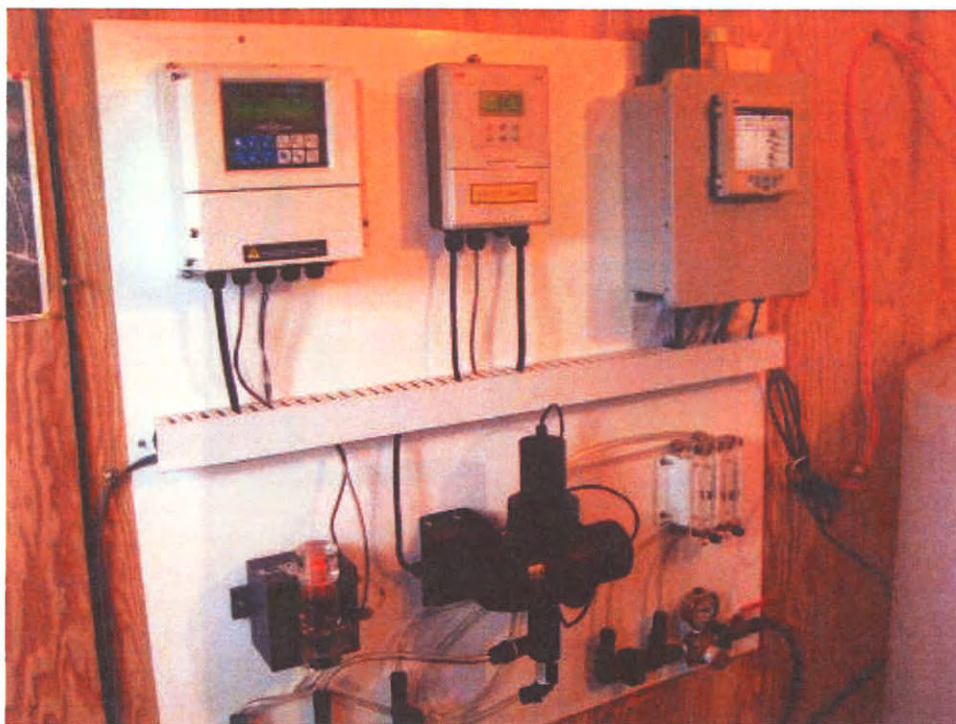
Photo 10: Chlorine Feed Controls
