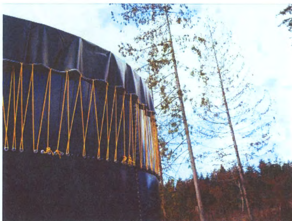
Photo 6: Bolted Steel Reservoir with Cover
