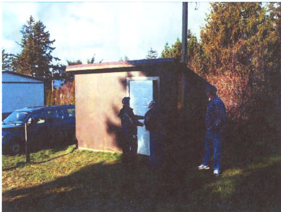
Photo 2: Well Pump Building
