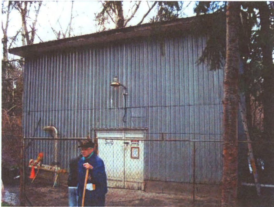
Photo 1: Booster Pump Station
