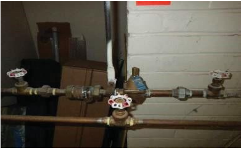
Copper piping with brass fittings and valves: Acceptable for continued use with monitoring for leaks. Presence of lead in solder and some fittings likely.
