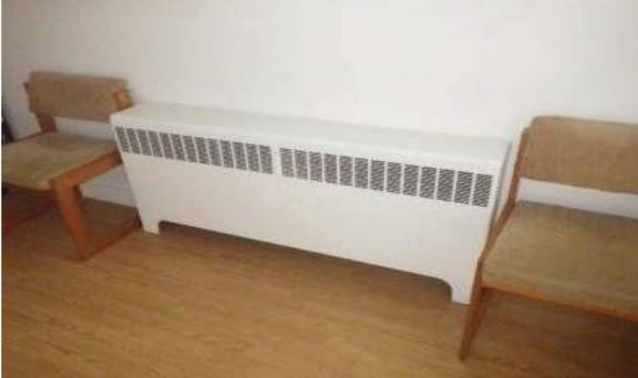
Hydronic convection heaters: Asset condition acceptable but will require significant renewal in the next five years for heating system reliability. Piping condition suspect in the absence of chemical treatment and corrosion inhibitors.
