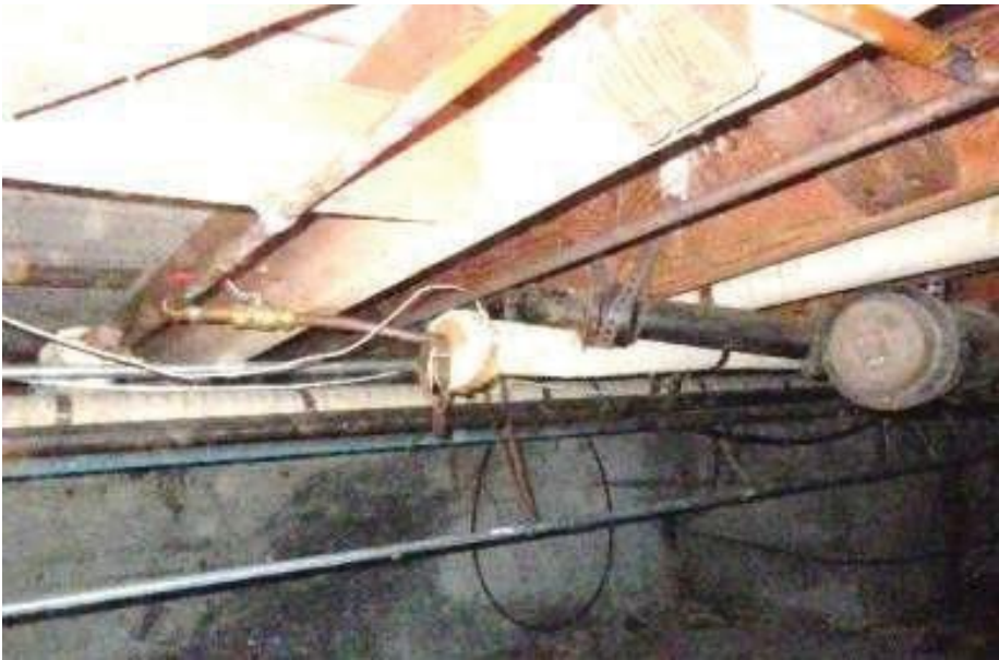
Cast iron and galvanized steel drain system with bell and spigot or threaded connections: Acceptable for continued use, but internal conditions likely deteriorating. Occasional jetflush cleaning and localized repairs may be required.
