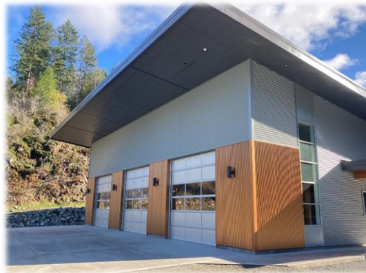
No.2 Fire Hall Built in 2020
