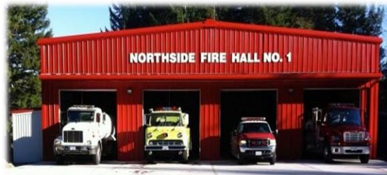
No.1 Fire Hall Built in 2012
