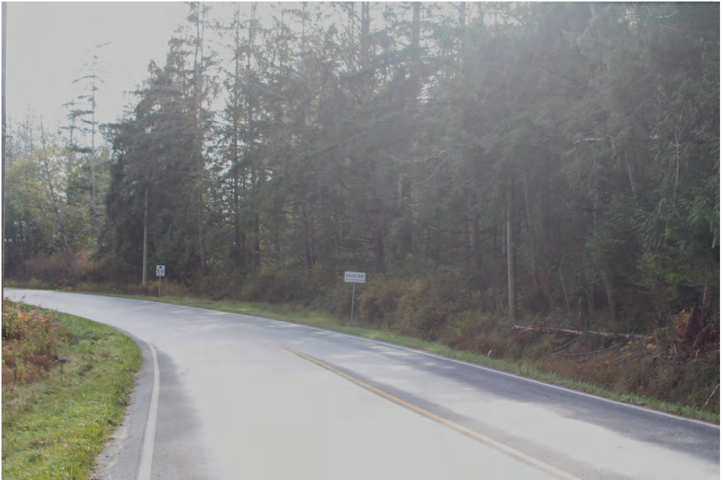
Northeast boundary of site (right) at Gillies Bay Road – Facing South
