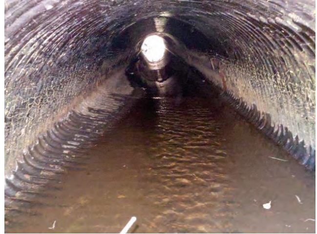
AREA 5 GILLIES BAY: ARCH PIPE (2256032) WITH LOCAL CORROSION
