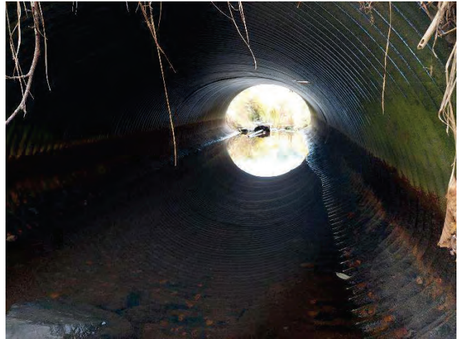
CULVERT 14 (3442927) INTERIOR: MINOR PIPE SEPARATION
