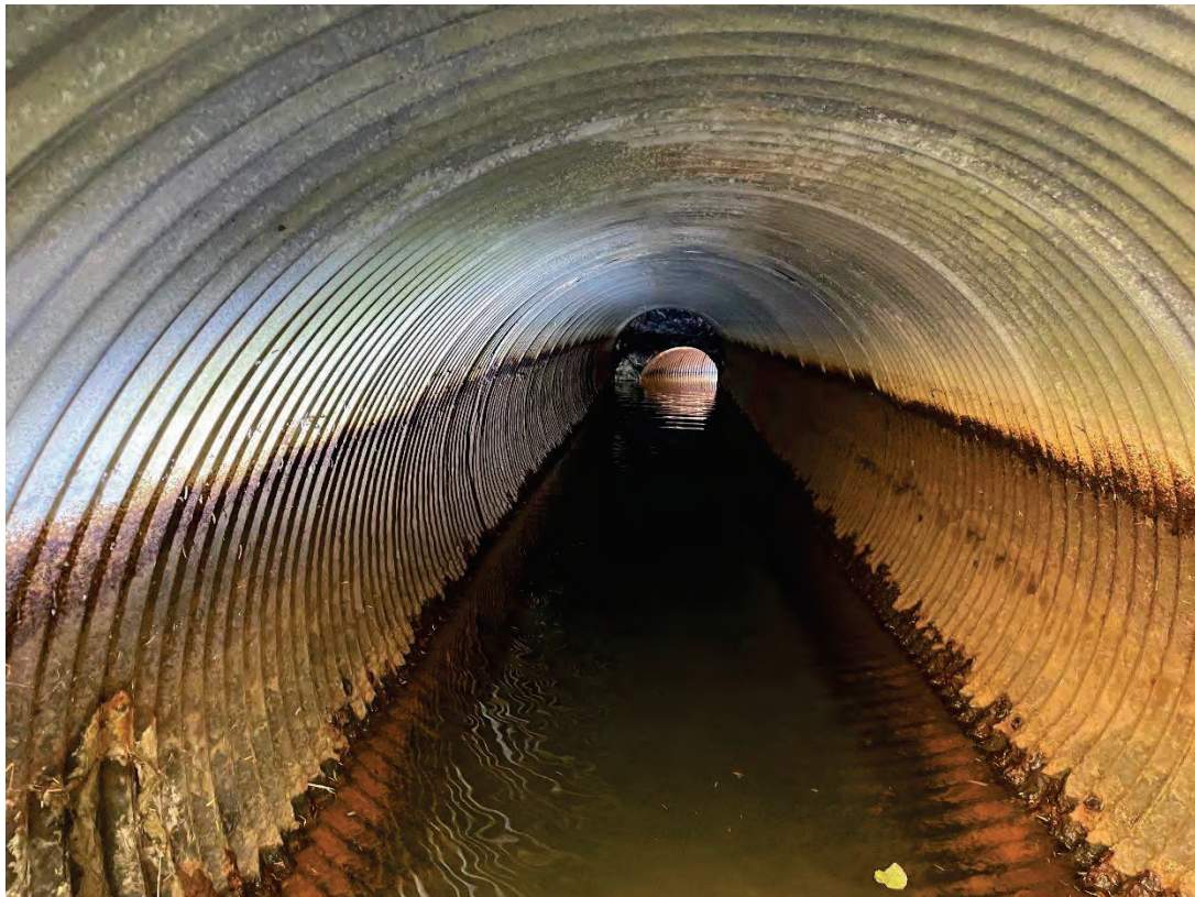
Pipe Interior facing DS: Pipe joint separation visible with skewed outlet pipe and visible rock
