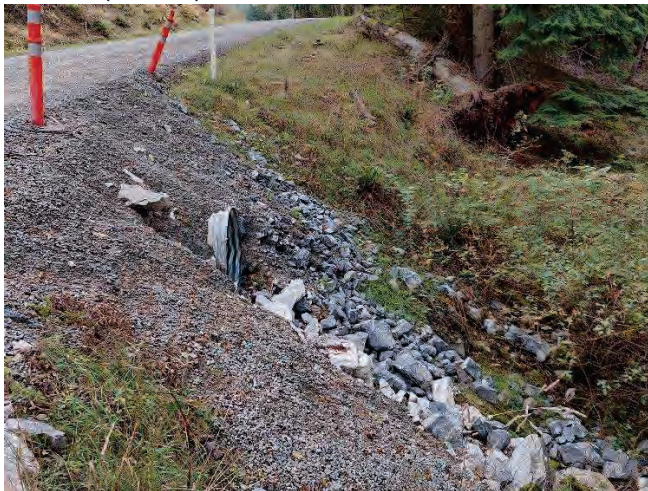
CULVERT 9 (2256424) INLET: WOODY DEBRIS AT INLET
