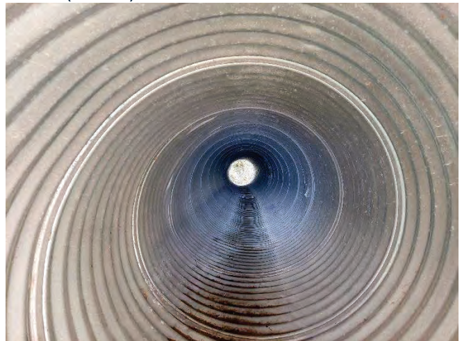
CULVERT 9 (2256424) INTERIOR: PIPE COATING MOSTLY INTACT
