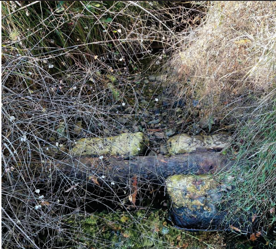
Upstream Channel facing US: DI utility service line visible in the upstream channel 3m from inlet
