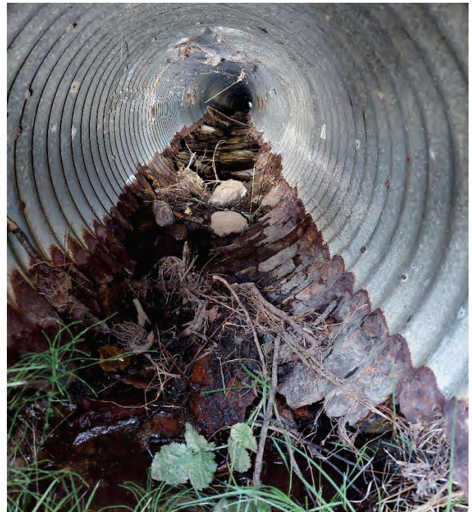
CULVERT 6 (2256019) INTERIOR: PIPE JOINT SEPARATION AND ROCK DEBRIS
