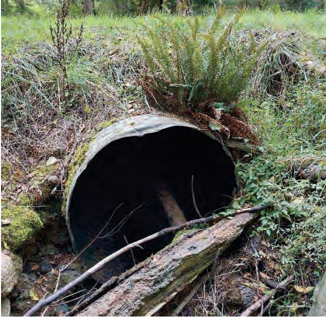
CULVERT 9 (2256424) INLET: WOODY DEBRIS AT INLET
