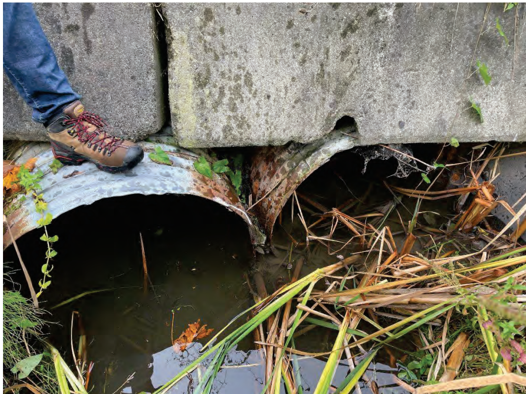
Culvert Outlet: Sediment Accumulation on right bank
