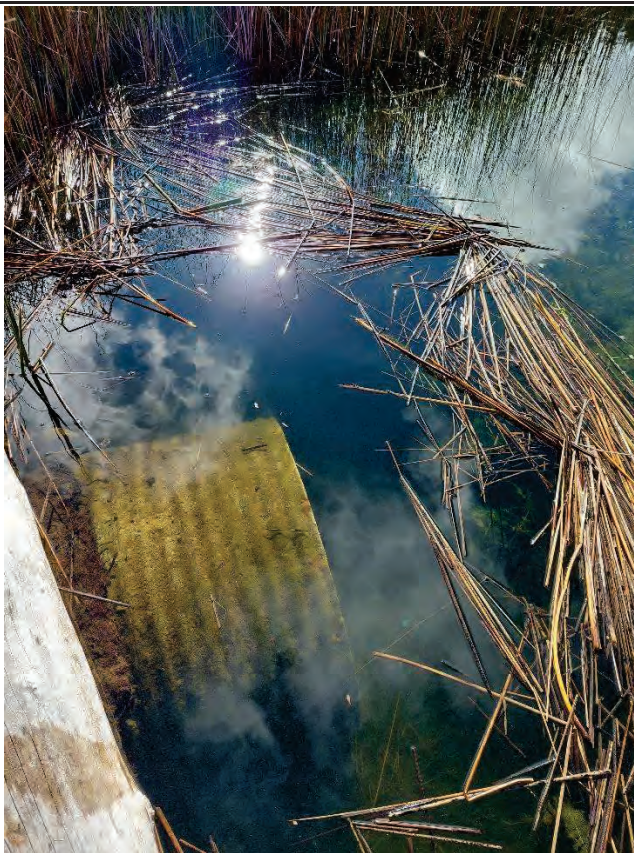
Culvert Inlet: Inlet fully submerged, log and reeds debris present above pipe
