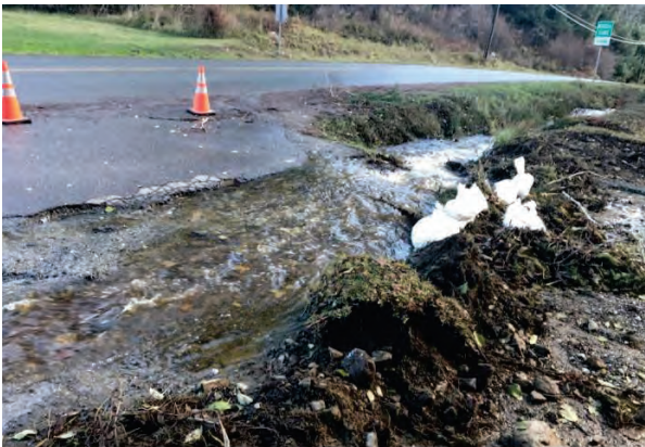
PHOTO 3: AREA 4 - OVERFLOW OF DRIVEWAY CULVERT (MOTI)
