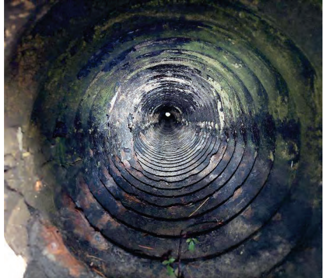
AREA 4 AIRPORT RD: 600MM CSP CULVERT (2256637) UNDER PINE ST INTERIOR, PIPE INVERT CORROSION
