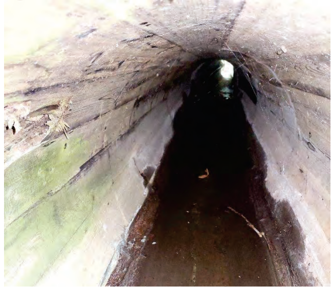
AREA 2 MARBLE RD: WOOD STAVE CULVERT (3442931) INTERIOR
