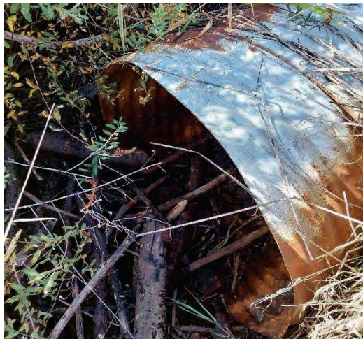
CULVERT 4 (2256045) INLET: MINOR WOODY DEBRIS
