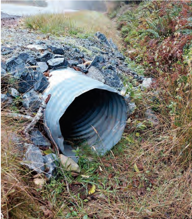
AREA 4 AIRPORT RD: NEW CULVERT INLET WITH IMPROVISED CHECK DAM INSIDE ROADSIDE DITCH
