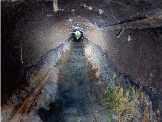
AREA 4 AIRPORT RD: 450MM DI CULVERT INTERIOR, SURFICAL CORROSION
