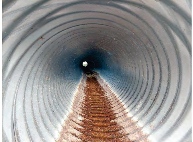
AREA 4 AIRPORT RD: 600MM CSP CULVERT (2256637) UNDER PINE ST INTERIOR, PIPE INVERT CORROSION
