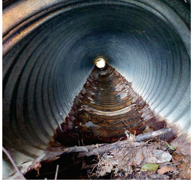
AREA 4 GILLIES BAY RD: OLD EASTERN 600MM CSP CULVERT, MAJOR CORROSION OF PIPE INVERT
