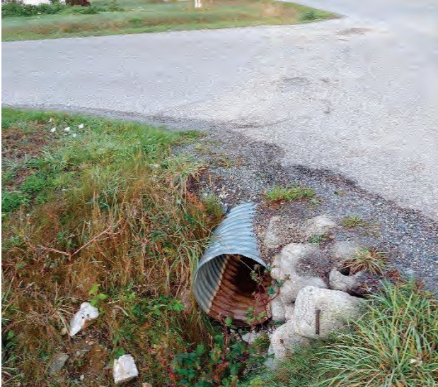
AREA 4 AIRPORT RD: 450MM DI CULVERT INTERIOR, SURFICAL CORROSION
