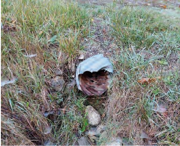
AREA 4 AIRPORT RD: 300MM CSP CULVERT (2258675) OUTLET, CORRODED INVERT
