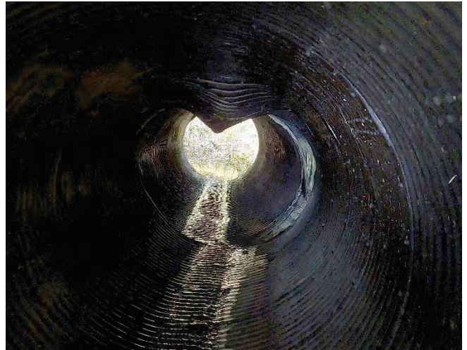
CULVERT 12 (2255061) INTERIOR: BUCKLING AND PIPE JOINT SEPARATION
