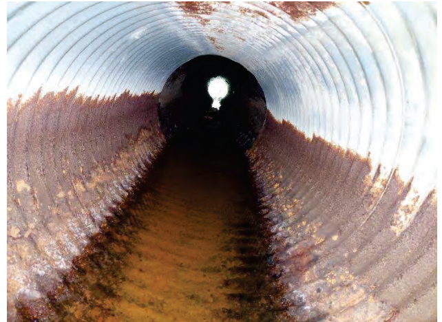
CULVERT 1 (2254949) INTERIOR: MATERIAL CHANGE AND HEAVY CORROSION
