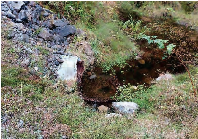
CULVERT 1 (2254949) INLET: DAMAGED INLET AND GRATE
