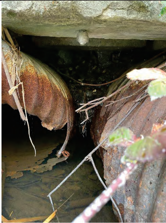
Culvert Inlet: CRB sitting on culverts, large cavity visible between twin pipes
