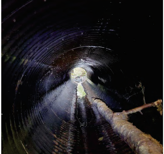
CULVERT 9 (2256424) INTERIOR: PIPE COATING MOSTLY INTACT
