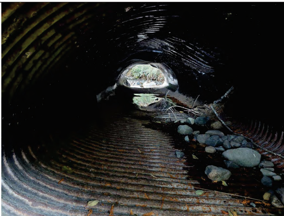
Culvert Interior facing DS: Buckling visible at 2 o'clock, flowing water visible in the middle of the culvert
