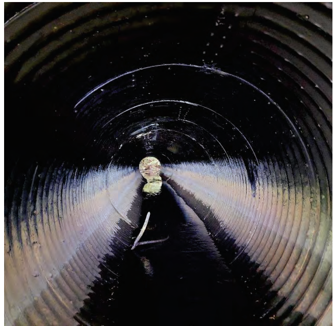
CULVERT 12 (2255061) INTERIOR: BUCKLING AND PIPE JOINT SEPARATION
