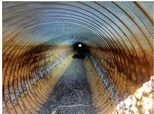
CULVERT 1 (2254949) INTERIOR: MATERIAL CHANGE AND HEAVY CORROSION
