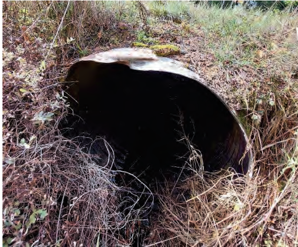
CULVERT 12 (2255061) INLET: INLET BEND
