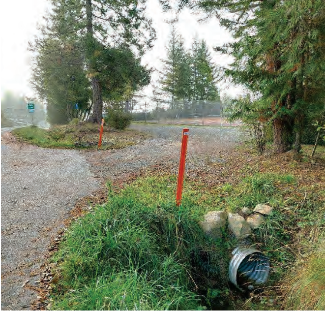
AREA 4 GILLIES BAY RD: TWIN 600MM CSP CULVERT INLET AT TENNIS COURT
