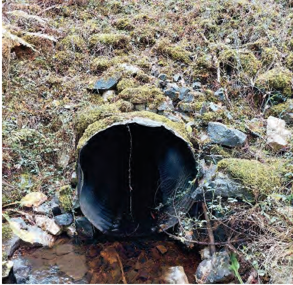
CULVERT 14 (3442927) INLET: PIPE COATING INTACT
