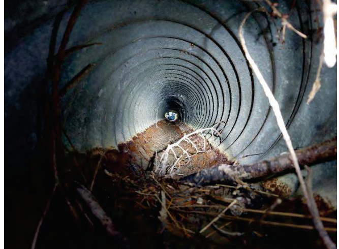
AREA 4 AIRPORT RD: 300MM CSP CULVERT (2258675), HEAVILY CORRODED INVERT
