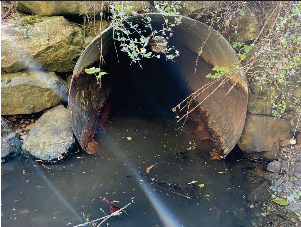
Culvert Inlet: Heavily corrosion at pipe invert with large section of missing material
