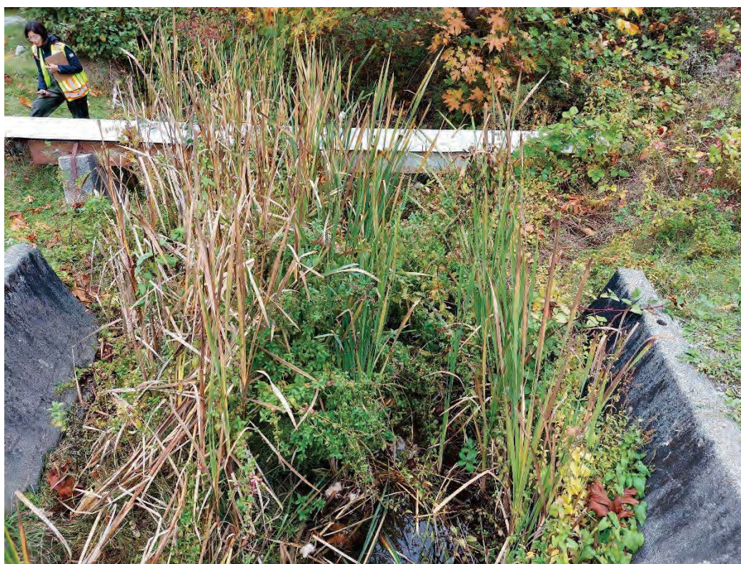
Downstream Channel facing DS: Sediment accumulation and vegetation visible & CRB wingwalls
