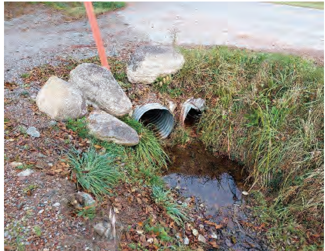
AREA 4 GILLIES BAY RD: OLD EASTERN 600MM CSP CULVERT, MAJOR CORROSION OF PIPE INVERT
