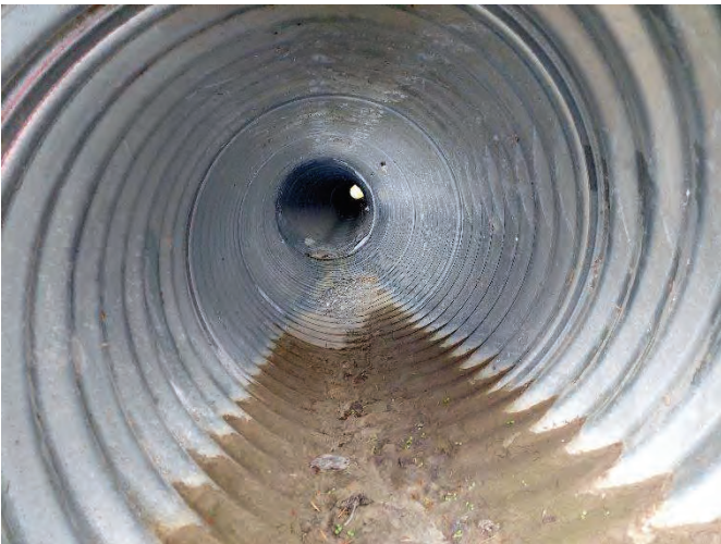
AREA 4 AIRPORT RD: NEW CULVERT INLET WITH IMPROVISED CHECK DAM INSIDE ROADSIDE DITCH
