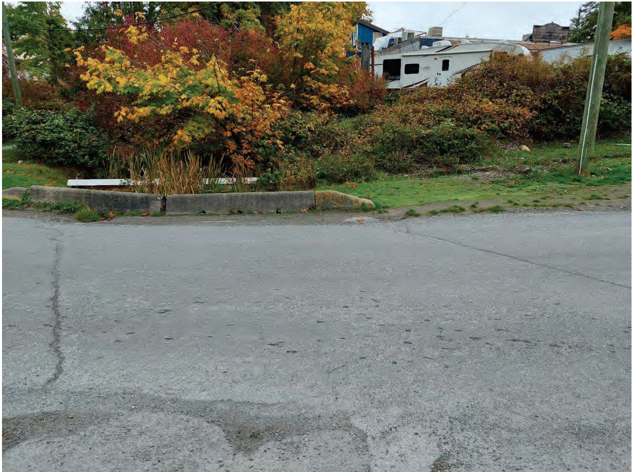
Pavement Surface: Tension cracks visible on the left and the right from the culvert crossing
