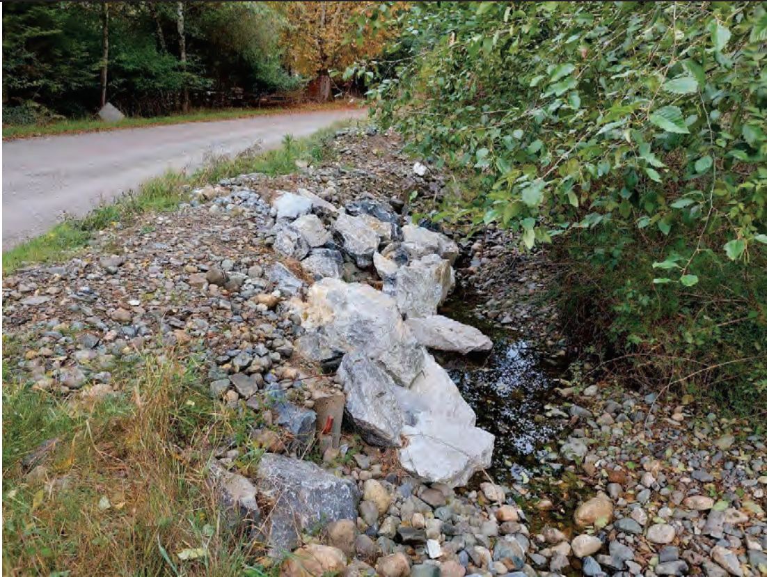
Upstream Channel at Bell Rd: Undermining of embankment along 14m stretch, dumped riprap visible
