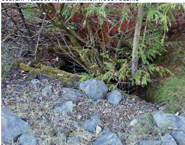
CULVERT 5 (2256047) INLET: VEGETATION PRESENT AT INLET
