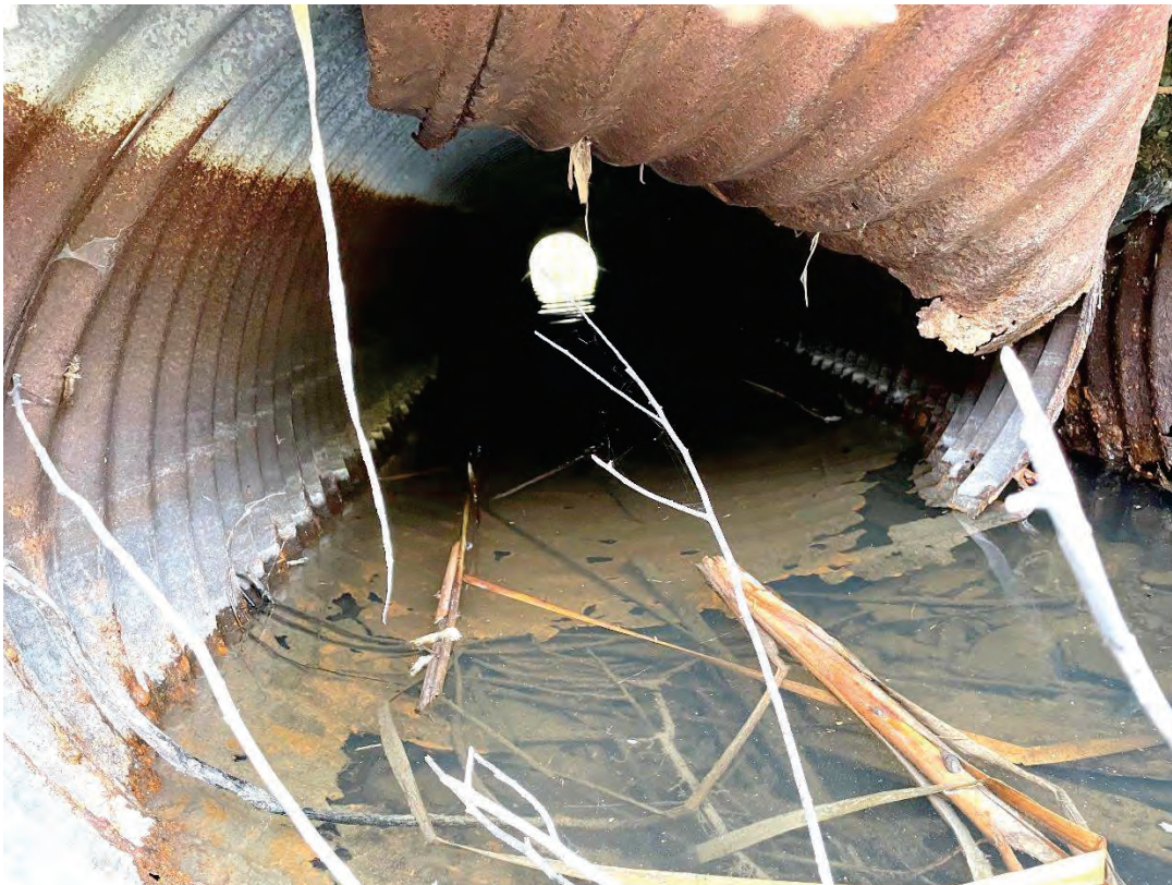
Pipe Interior (western pipe) facing DS: Visible damage of inlet and heavy corrosion of invert
