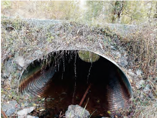
CULVERT 14 (3442927) INLET: PIPE COATING INTACT
