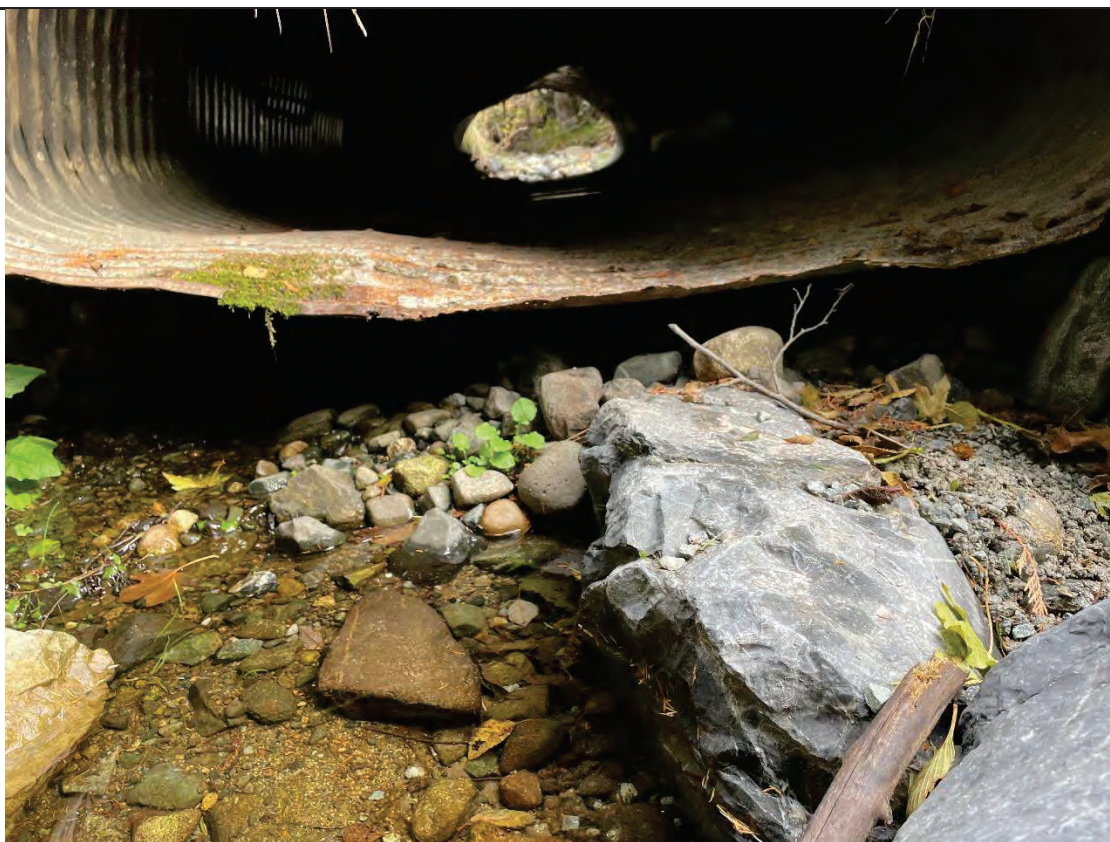
Culvert Outlet: Visible undermining of culvert pipe with visible stream flowing under pipe
