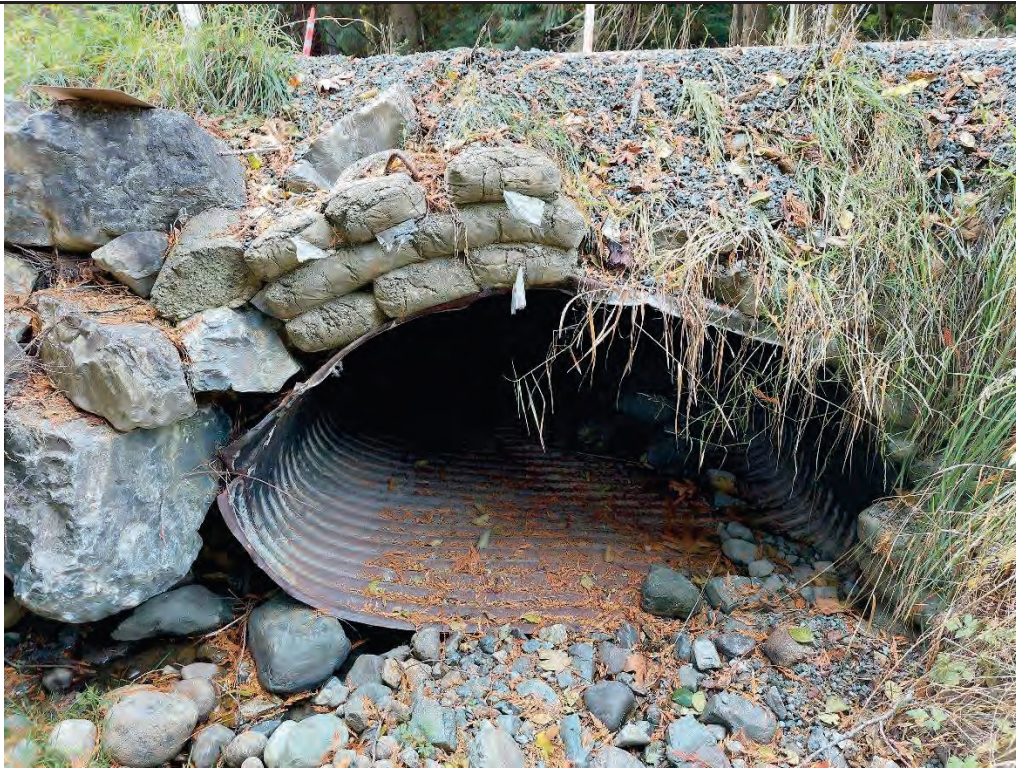
Culvert Inlet: Failed concrete bag headwall, culvert pipe visibly corroded, flow below gravel
